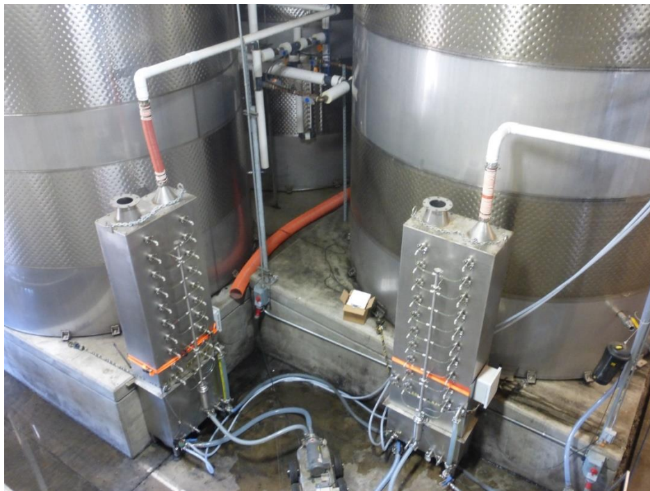
NoMoVo control systems (2)
